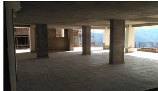
Ample Covered Parking in Stilt Floor in Block B
